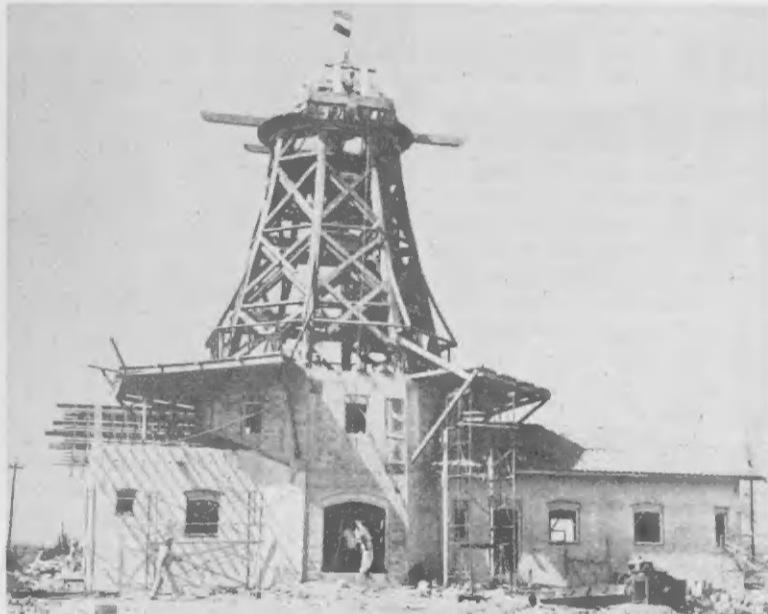
A NEW foundation, its architectural lines complimentary to the old mill's lines, supports the 147-year-old structure. UN FUNDESHI nobo, su linjanan architectural complimentando e linjanan di e mulina bieuw, ta wanta e structura.
